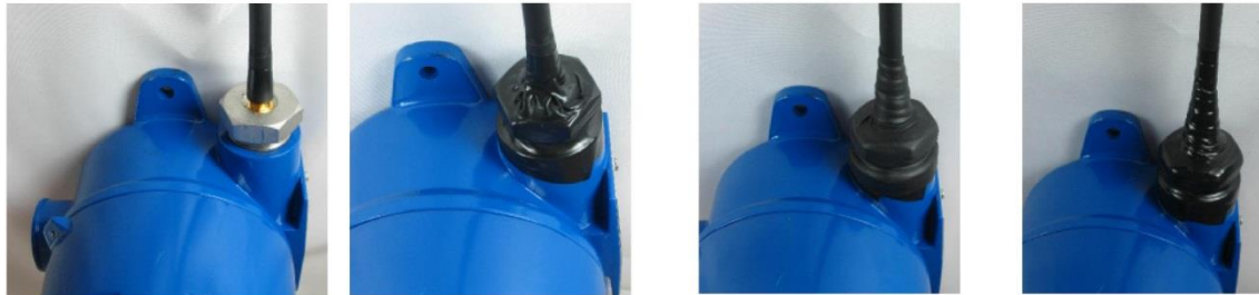
Figure 4-4 Water Proofing Antenna Connections
